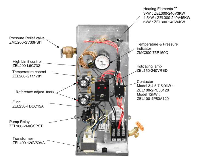
\*\*When replacing an heating element, insure that its orientation is identical as the original
